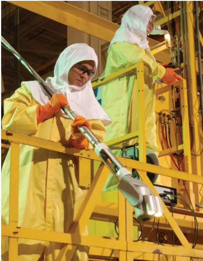
Operators perform nuclear reactor vessel visual inspections with Ca-Zoom PTZ Digital Inspection System
