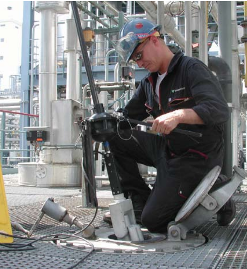
Inspecting chemical plant vessel with PTZ140 system, extension pole and swivel ball tripod.
