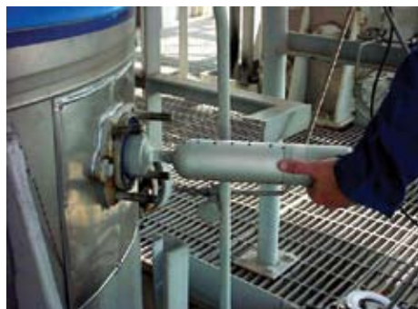
Glass-lined vessel inspection through Pharmaceutical tank inspection through 76 mm (3.0 in.) nozzle
