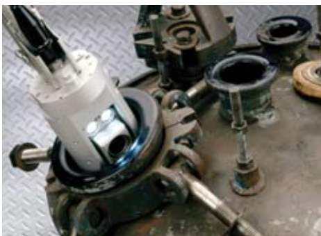
Inspection through a 100mm (3.94 in.) \varnothing nozzle
